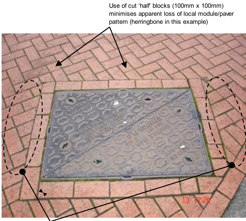
Figure NGA12.4 Acceptable Loss of Module Pattern - Modules up to 300mm [Picture 1]
